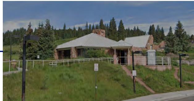
Current Rest Area Site and Building
